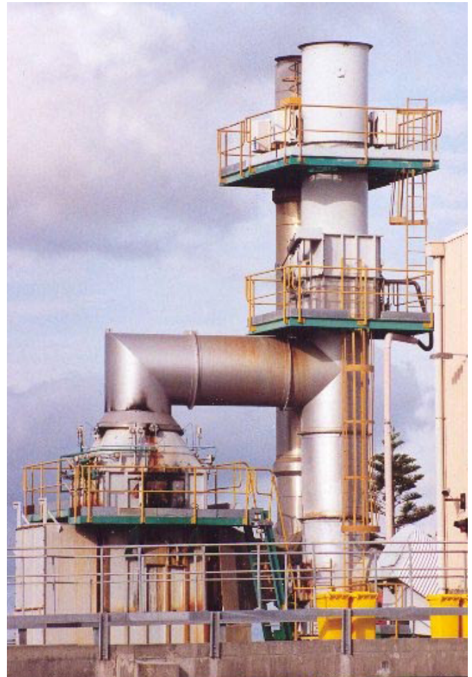
The old Auckland Airport Incinerator stack.
